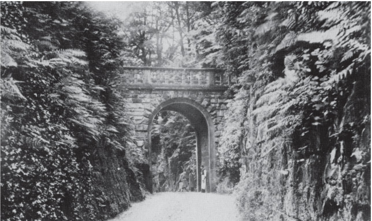
FIGURE 16. The Gorge, leading from hall to stables, was cut through a ridge in 1833. The walls are of Keele sandstone, partly natural, partly built up. The near section was refaced with Macclesfield stone in 1962. The original ornamental stone balustrade of the bridge was replaced with brick about 50 years ago.
