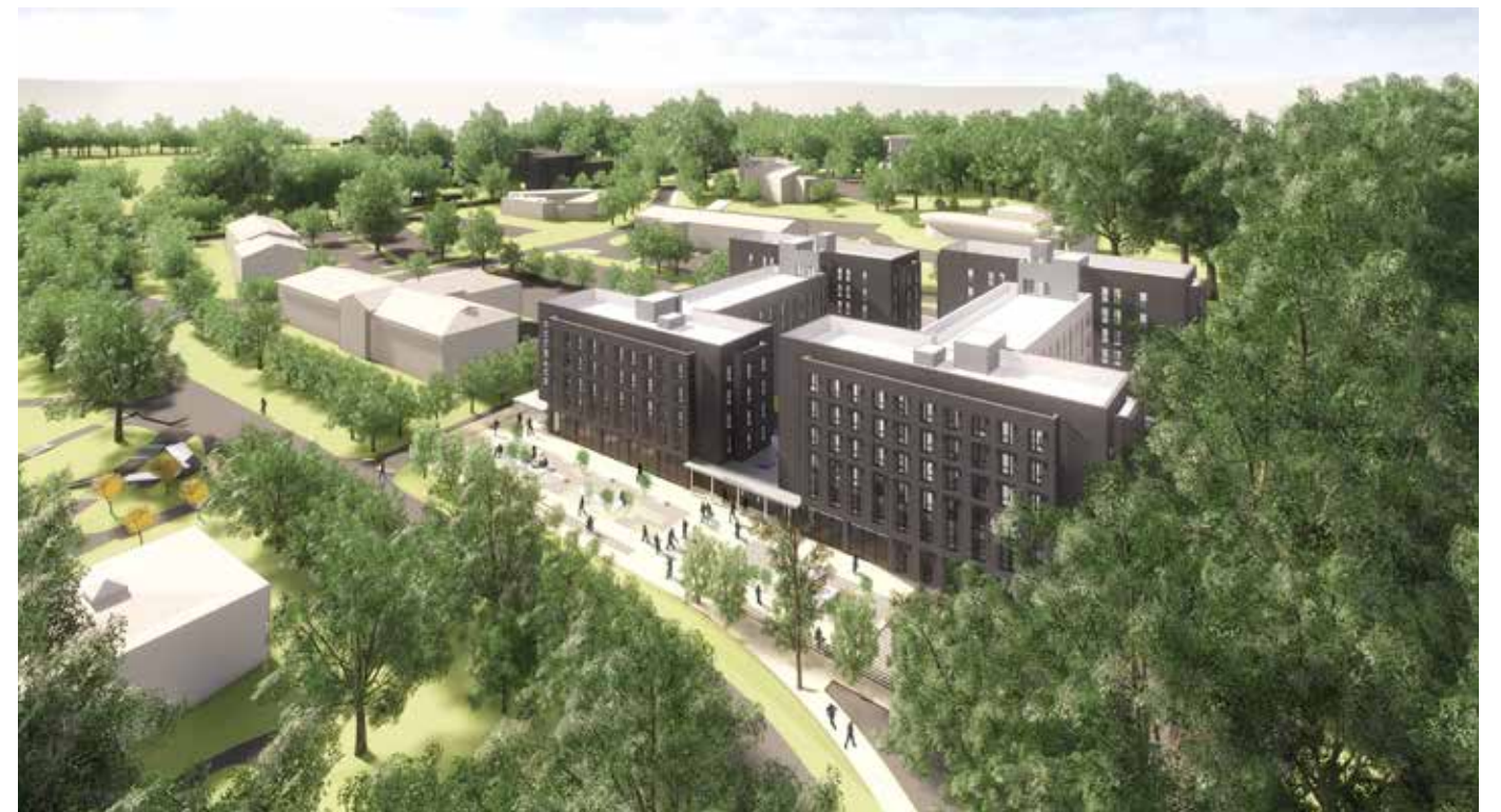
Horwood A&B aerial view
