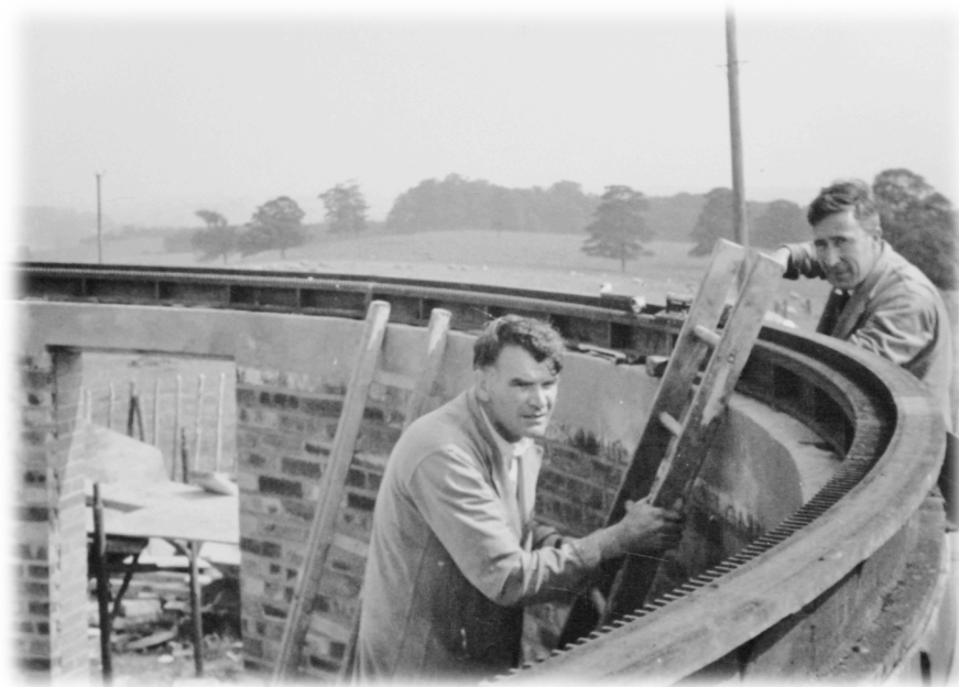
Figure 4 Leveling the base ring at the Keele site. Harry Wardell of the University Workshop on the ladder.
