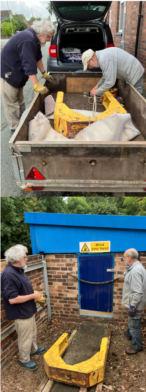
Figure 4 Doody's mount's fork, lifted and laid to rest.
