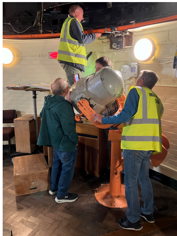
Figure 3 Paul Klimczak working on the dome rail (with mains power switched off) while others look on.
