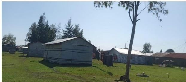
8 - Displacement due to floods necessitating move to camps/temporary accommodation with limited amenities
