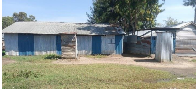
9 - Displacement due to floods necessitating move to camps/temporary accommodation with limited amenities
