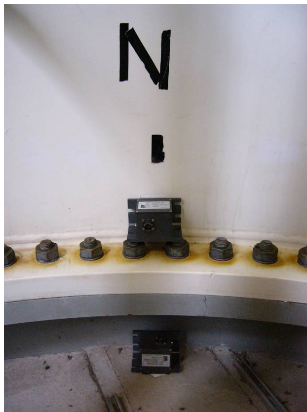
Figure C4 CMG-5U sensor showing positive acceleration direction
